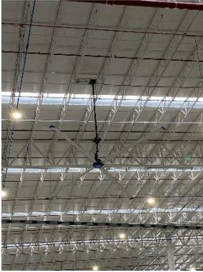
**Monterrey ceiling:** The ceiling of Genie's newest manufacturing facility in Monterrey, Mexico includes fans to help with cooling and air movement, panels that let in natural light, and LED lights that feature sensors to adjust to what is needed in addition to what the natural lighting provides, all of which helps use electricity.
